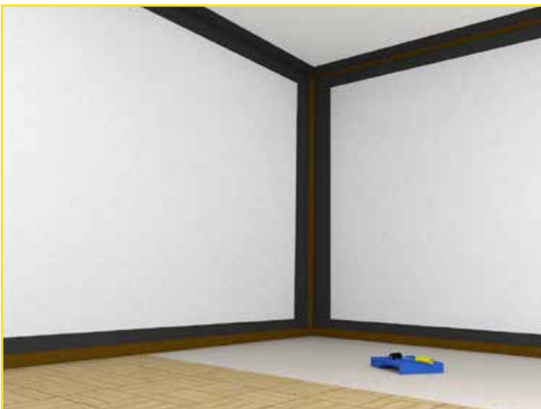
Fig.5: First painting of the room corners, window reveals, and the areas concealed by the heater.
